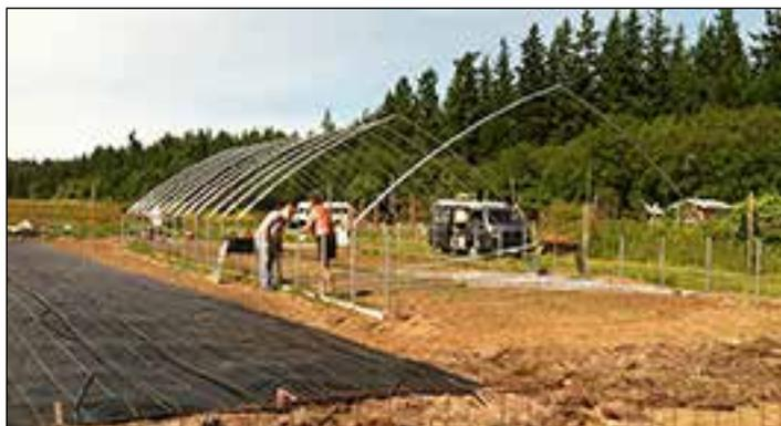
The hoops are being mounted on carefully placed metal poles, so they slide right on. Dorcas Young's helpful contractor neighbor, Tom, set the corners and positioned the poles. With Lynae Slinden's help, the hoops have been mounted.
